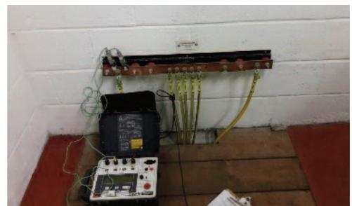
Bonding measurement performed onto Substation Earth Bar
